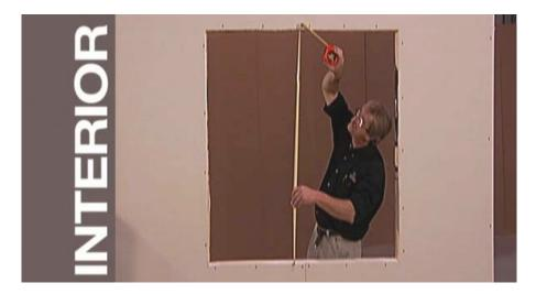
Check the sill for level. Use a properly sized level when checking the sill for level.
