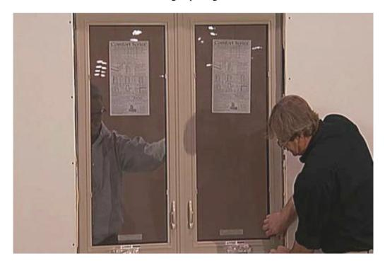
When lifting the window into the opening, use caution by making sure the window is fully supported at the sill, so that damage from the stress of lifting the window will not occur. Always lift the window in an up-right position. **Lifting the window in a flat position can cause damage.** The window should be lifted into position and set onto the shims with equal spacing from each jamb.
