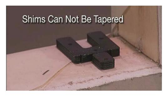
Once shims have been placed on the sill, check for level again.
