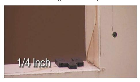
Horizontal sliders will require shims to be placed 2" in from each jamb and under the mullions.
