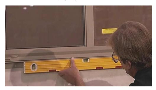
Then check the gap on both sides from the inside of the window.
