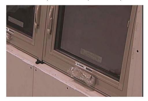
Do not use shims under the center of the single hung or double hung window. Note that the shipping and installation strap that the factory installed on the double hung must stay attached until the installation is complete.
