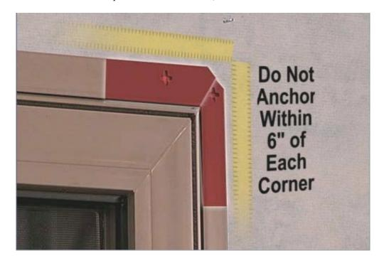
The nails must be centered in the star hole with a snug fit.
