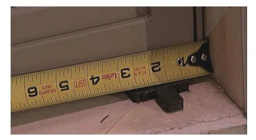
The shims used at the sill for leveling the window cannot be tapered. The window must be able to be set flat on the shims.
