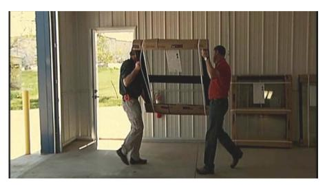
When Comfort Series windows are ordered as rough opening sizes, Gerkin will down size the windows 1/2" smaller than the rough opening sizes given. This reduction in size gives the window sufficient tolerance for proper shimming and insulating. Comfort Series windows can also be ordered as exact window dimensions for a more custom fit.
