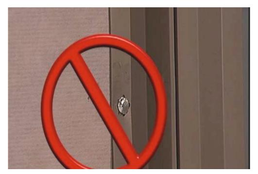
Do not pull down on the window head while nailing the head, as this could sag the head prior to nailing.
