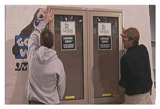
Once the window is in the rough opening, check the window to make sure it is level.
