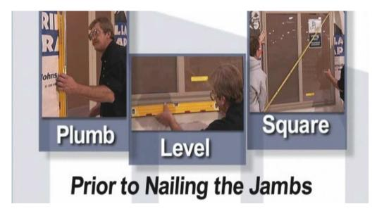
Once the window has been properly positioned, place a 2" roofing nail near the center of each jamb.
