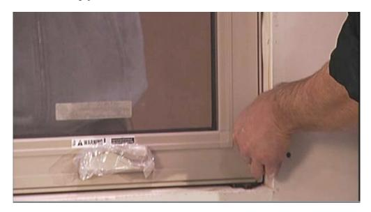
Check for square. To do this, you should measure diagonally from corner to corner on the window frame as well as the sash opening.
