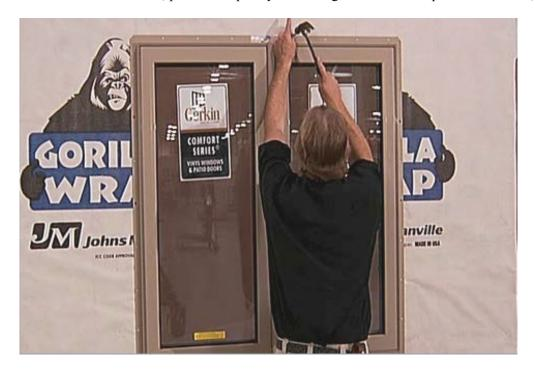
then secure the sill with 2" roofing nails through the center of the star holes.
