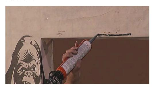
The centerline of caulk should be about 1/2" from the edge of the rough opening.
