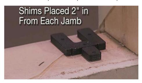
Single hungs and double hungs will require shims to be placed under the jambs.
