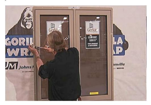
Re-check the jambs for bowing as well as square and plumb.
