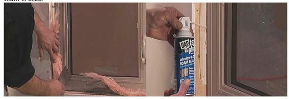
Gerkin recommends the use window wrap tape over the nail fins of the window. Apply tape to the sill first, then the jambs, and finally the head.
