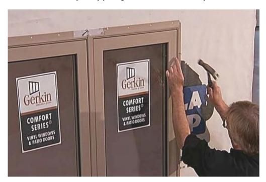
In order to allow for expansion and contraction, do not anchor within 6" of each corner.
